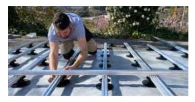
Low double joist 15,5 x 54 mm
